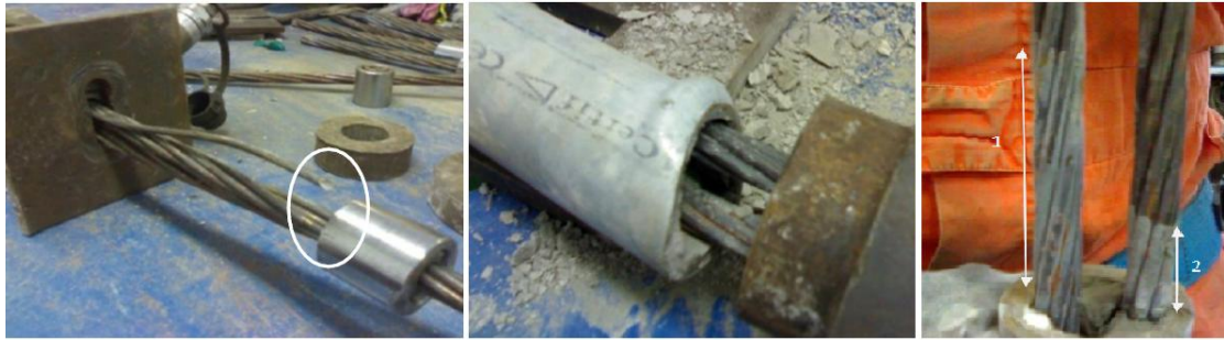
Figure 4.4 – Cable strand rupture (left); Steel pipe deformation (centre); Displacements: 1- displacement of the pulled cable, 2- displacement of the other cable (right).
