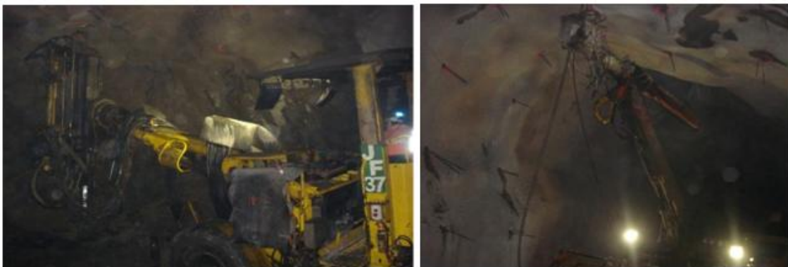
Figure 4.1. – Drilling operation (left); Cables application (right).
